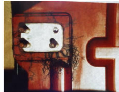
This dangerous tracking was located deep within the switchgear.
