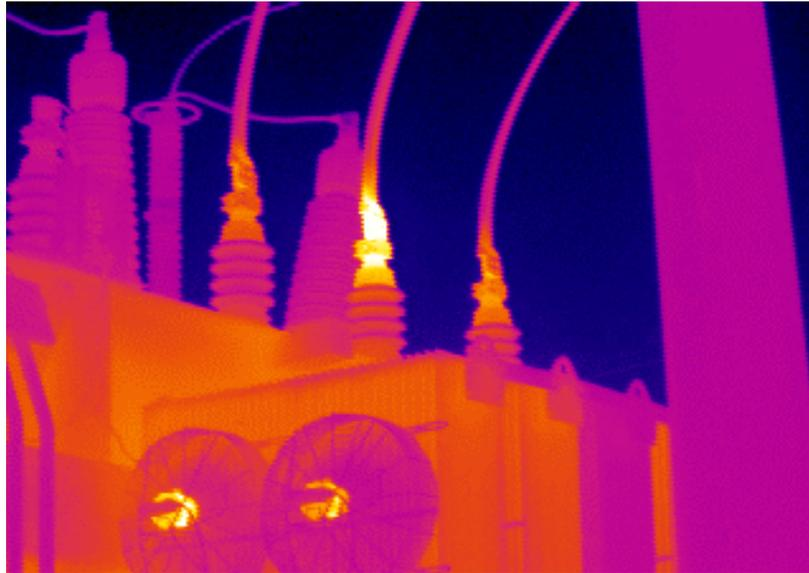
***This infrared image shows heat build-up on the center-phase secondary bushing connection on an oil-filled transformer. The use of infrared technology prevented a catastrophic failure from occurring.***
