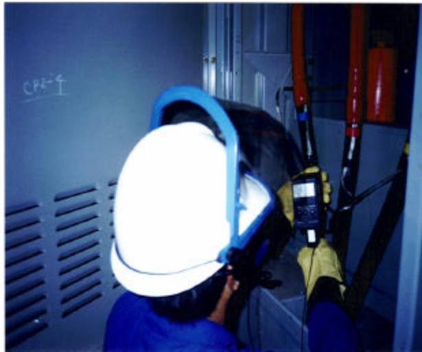
***Photo of a technician performing a field partial discharge survey of a medium voltage cable. The technician safely applies the sensor to the grounded cable shield while the electrical system remains in service.***
